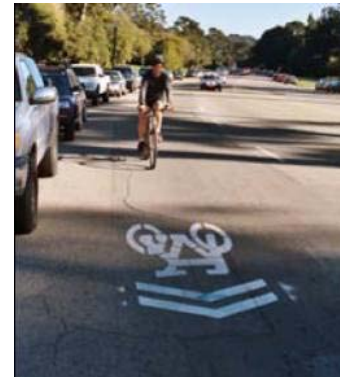
Sharrow Pavement Marking
